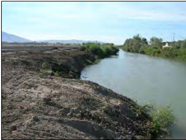
Midvale site riparian forest complex restoration recontouring on the Jordan River.
